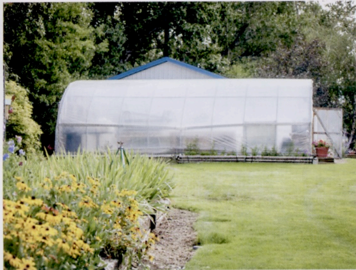
The non-profit organization Jackson's Garden obtained help from the USDA Natural Resource Conservation District to build a high-tunnel greenhouse to extend the limited Montana growing season. (Photo by Sara Gilman)
